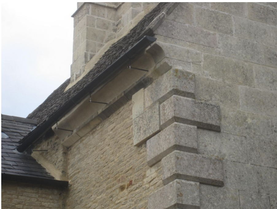
Detail of south-west corner, with eaves cornice running up to offset
