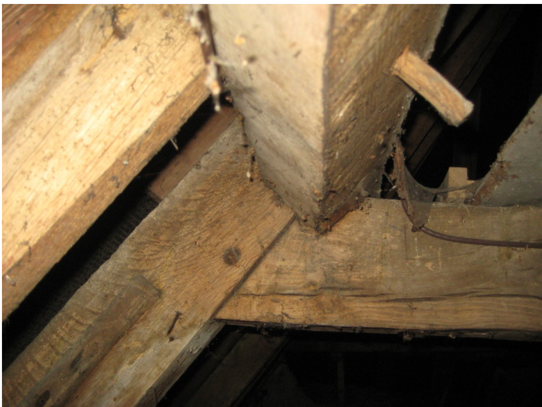
Clasped purlin truss to main block
