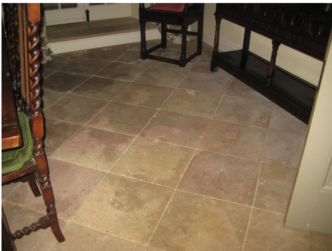
Ketton stone floor to central room
